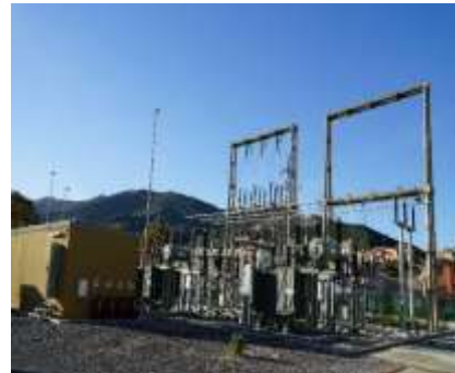
132 kV substation
