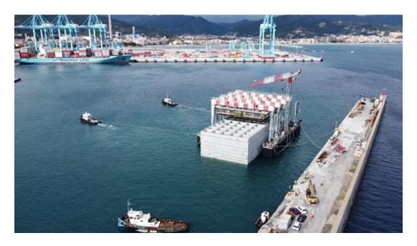
It ranks as the largest caisson to have been constructed to date with this range of equipment by Fincosit, pioneers of the industry: up to 25.6 metres high, 31 metres long, 22 metres wide and weighing up to 9340 tons. The reinforced-concrete cellular caisson was precast on the floating dock Dario, deployed by the company at the service of the breakwater extension in the Port of Vado Ligure.
