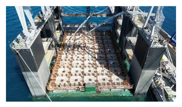
The New Open-Sea Breakwater takes shape as the fast-paced construction of the caissons takes off, with the near-completion of the first of 100 caissons set to form the 6,200 metre port facility.
