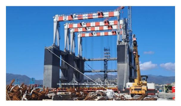
The construction of the first of 100 caissons, which will form Genoa's New Open-Sea Breakwater, takes shape on board the "Dario" floating dock positioned in the Port of Vado Ligure.
