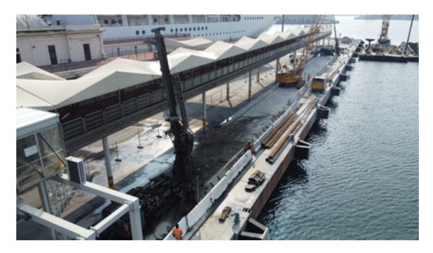
The construction works at Genoa's cruise terminal press ahead as jet grouting operations are underway in the final phase of the retrofit and renovation of the Ponte dei Mille western quay wall.
